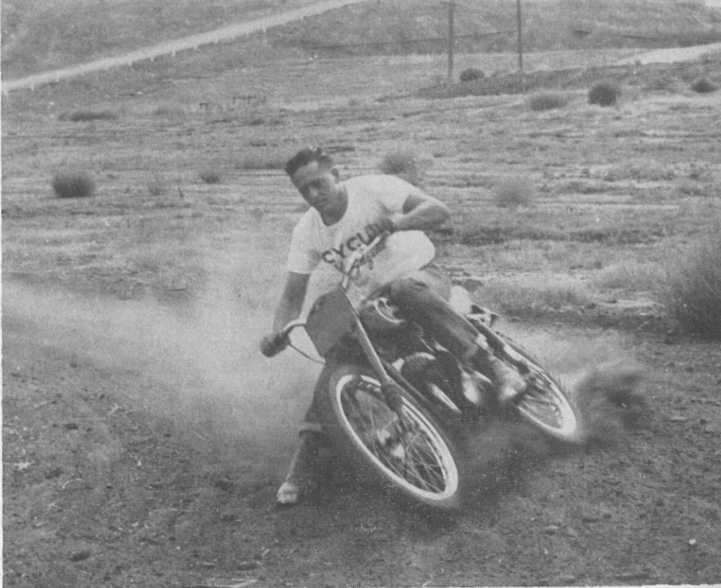
Handling quality of the James was excellent. Here the little bike is put to the test in a series of severe slides in soft rough dirt. No tendency to bounce was noticed and weight distribution seemed ideal.
